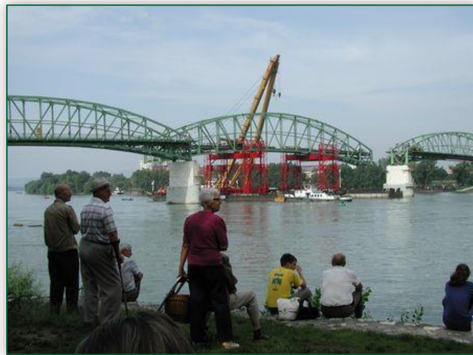
Figure 4: Mária Valéria Bridge under reconstruction
