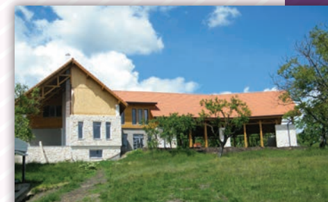
Training centre under construction in Răscruci
